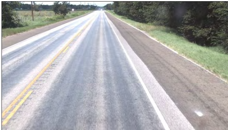
Figure 35. Photo. Chip seal road with raveling at MM 480 (SR30 = 32.5, MPD = 0.88).
